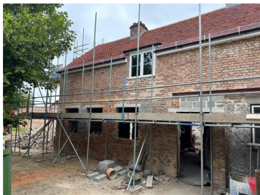
Main entrance with new roof
