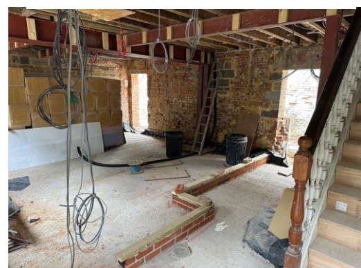
Science Lab with openings to Prep Room and offices
